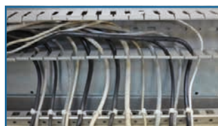
Cable Fixing Cross Members
